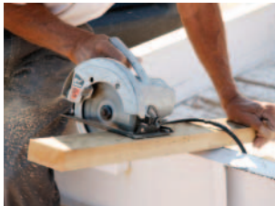
Construction Site Application
